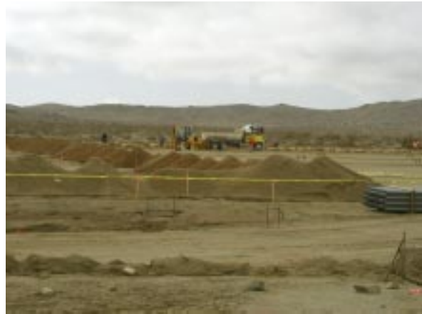
Solar Field under construction 2-25-04
