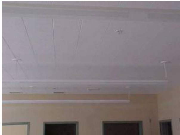
Ceiling tile and light bars in Adjunct Faculty office area.
