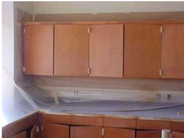
Cherry staining in process on the cabinets in the Office Service Area
