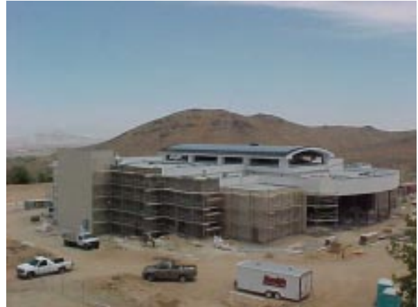
West elevation, EIFS finish complete on roof walls, stone veneer complete.
