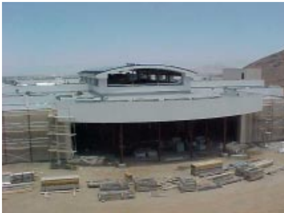
South elevation, EIFS finish is installed and scaffold is coming down.
