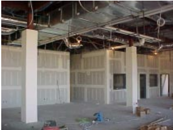
1st floor gyp. board and taping continues.
