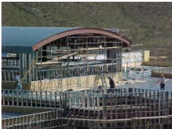
Carpenters are installing exterior plywood at roof parapet walls.
